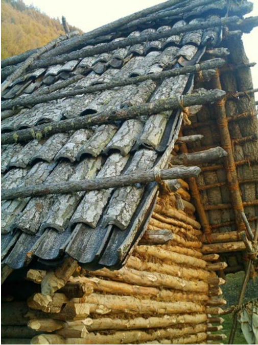
Fig. 16: Thatching of a Neolithic house model with lime bark shingles, alternating upside and downside, ArcheoParc Schnalstal (Italy)
