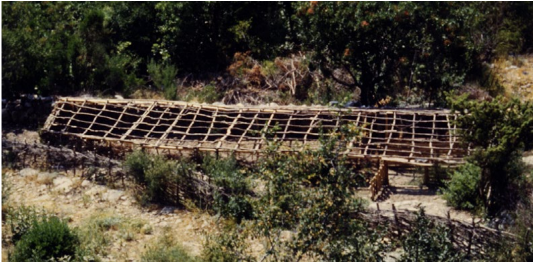
Fig. 14: Barn construction site in Anatolia. Photo: Lothar Breinl
