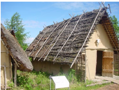
Fig. 15: Thatching of a Neolithic house model with lime bark shingles, Federseemuseum Bad Buchau (South Germany)
